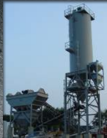
115 COMANCHE BATCH PLANT 720 ARROWHEAD SILO
