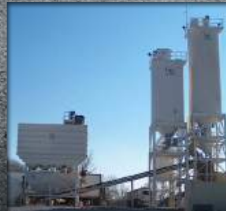
APACHE BATCH PLANT 943 ARROWHEAD SILO & 720 AUXILIARY SILO
